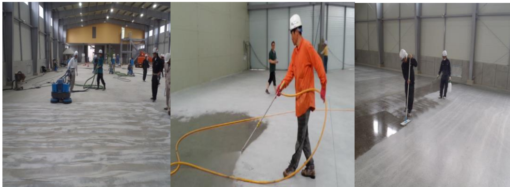
< Concrete Hardening Procedure >
