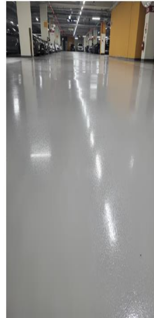
Sporthane KS Hyper Floor applied in an underground parking lot
