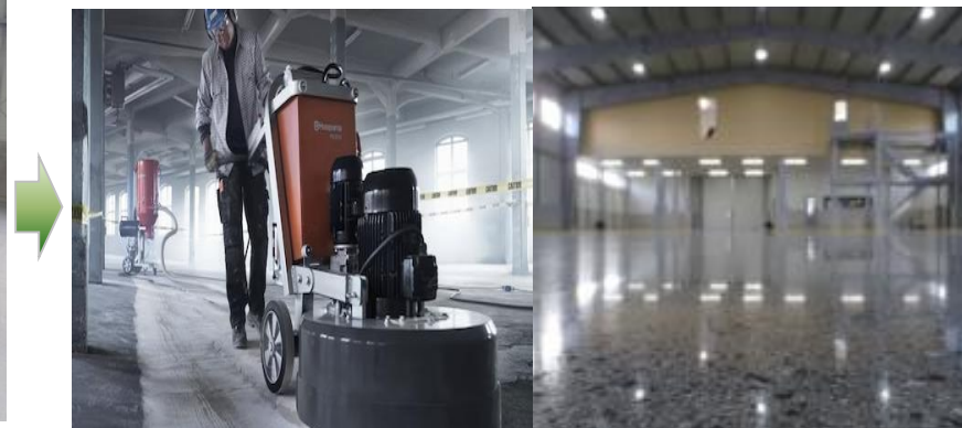
< Concrete Polishing Procedure >
